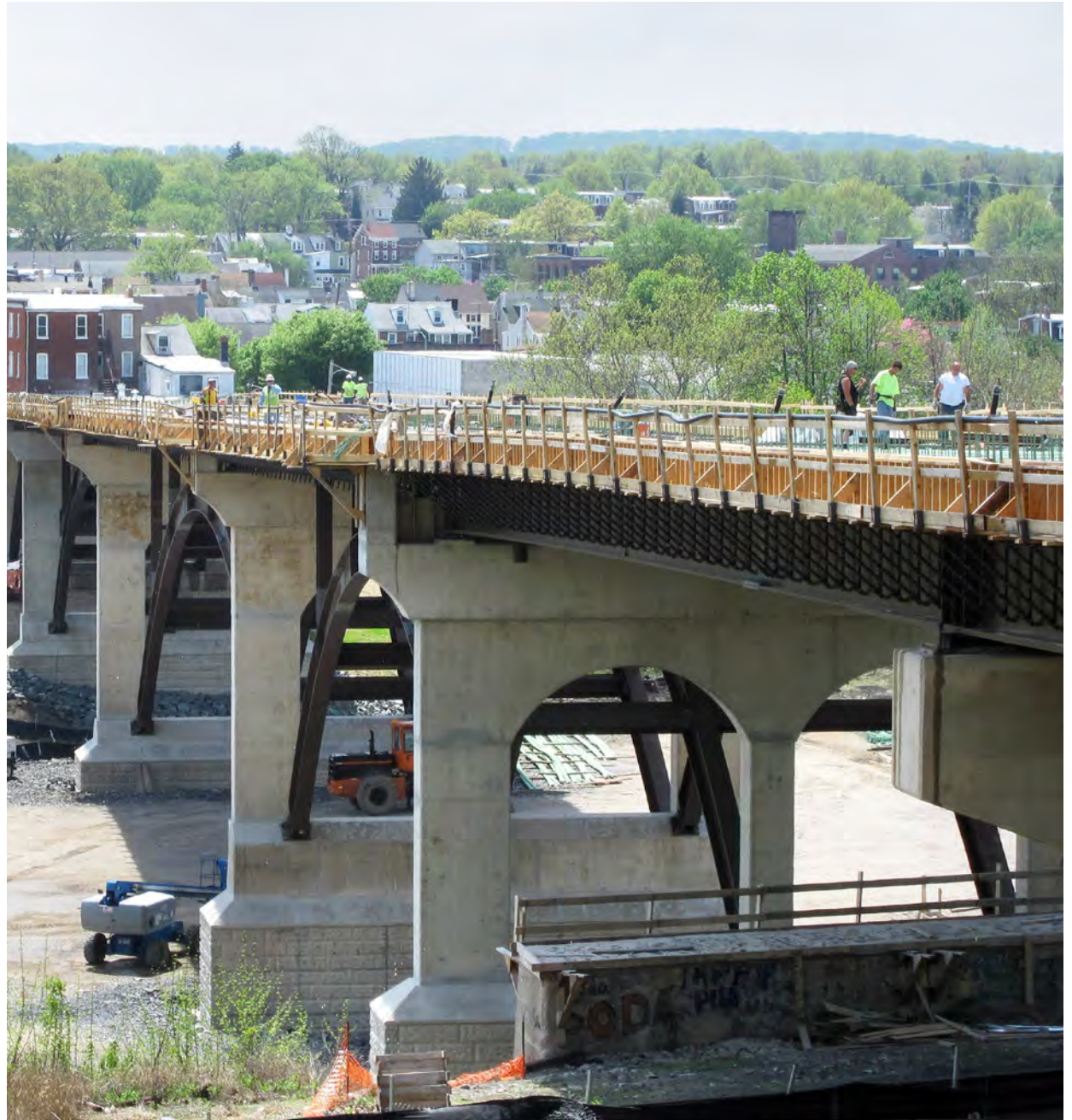
Construction of the Gay Street bridge in Phoenixville.
