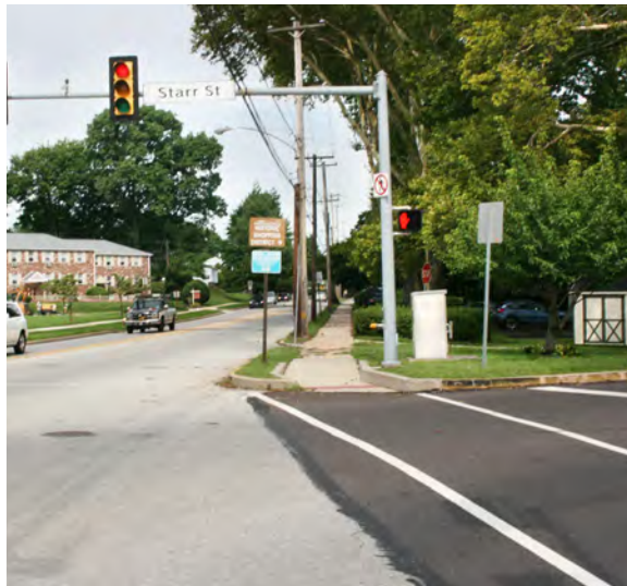
A crosswalk, pedestrian walk signal, and ADA curbing at the intersection of Starr and Nutt Road, Phoenixville.
