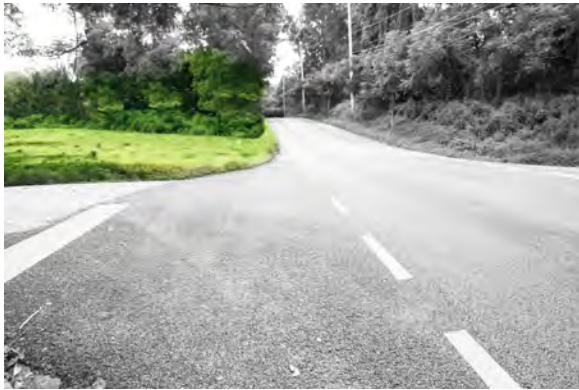
Pavement markings would help alert drivers to the intersection.
