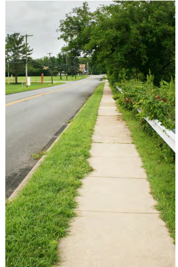
Sidewalk on Charlestown Road in Schuylkill Township.
