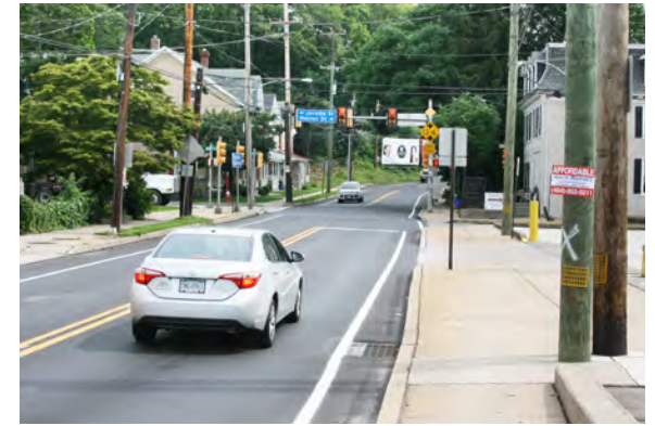
Looking north on Bridge Street Towards the Jacob and Walnut Intersection to be realigned.
