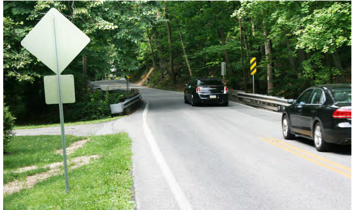
View north along PA 29 towards existing one-lane bridge, approximately 300 feet north of the Union Hill Road intersection.
