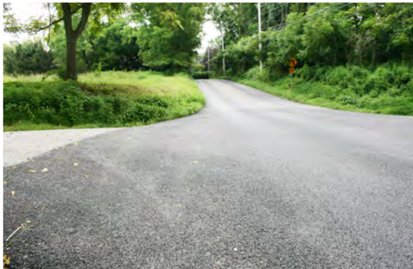
Existing view south toward Charlestown Road and Hollow Road intersection. Note the existing high friction pavement surface in the foreground.
