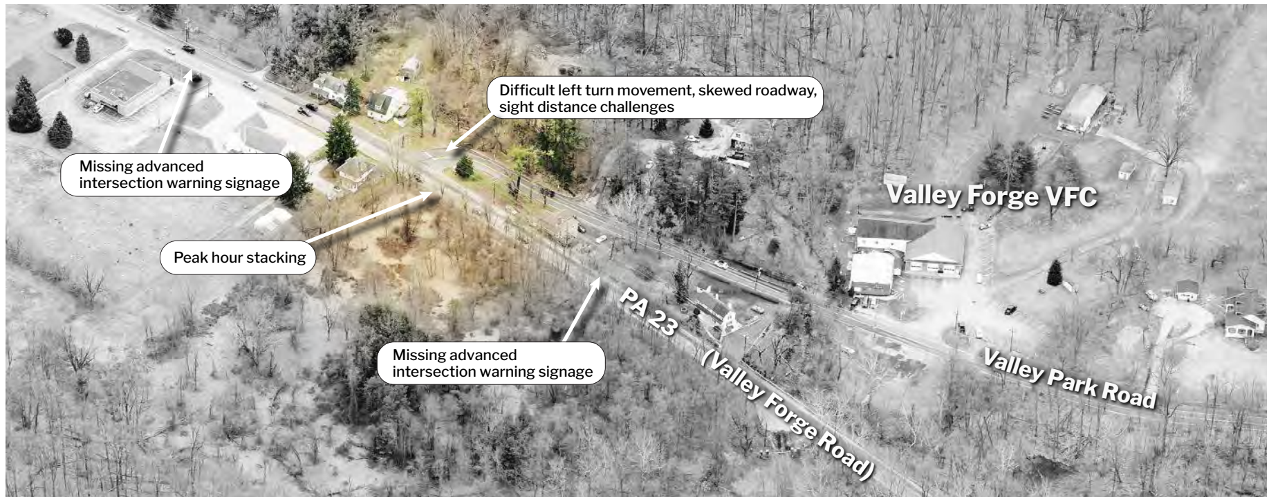
Existing conditions at the PA 23/Valley Park Road intersection. Source: Pictometry.
