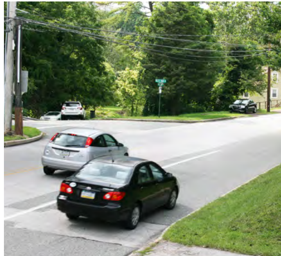
Existing PA 23/Valley Park Road intersection.
