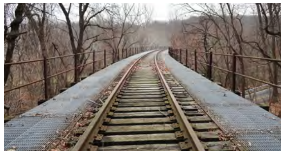
The impressive 600 foot long, 50 foot high trestle over Pickering Creek and State Road in Charlestown Township. Image credit: Campbell Thomas and Company.
