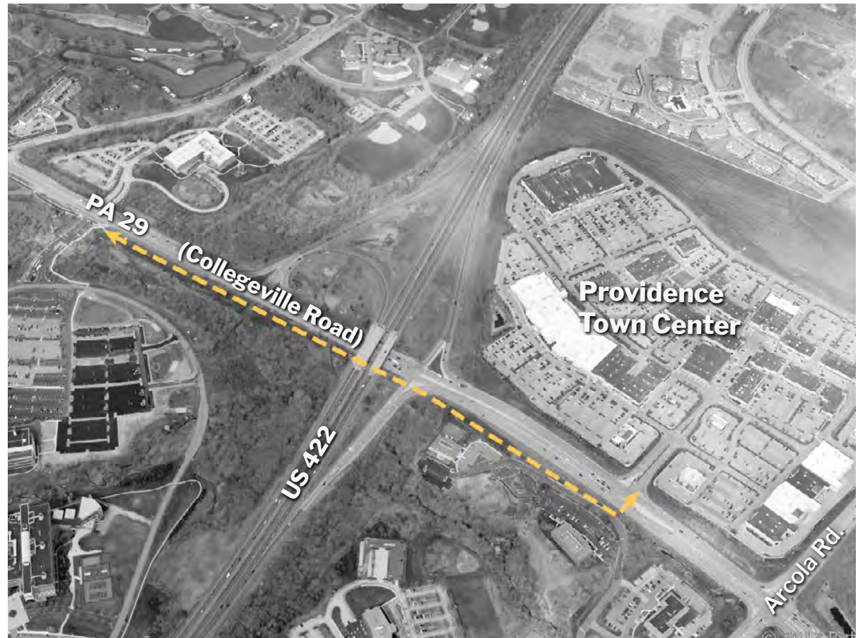
Aerial view toward the west of the PA 29 and US 422 interchange and surrounding area. Source: Pictometry.
