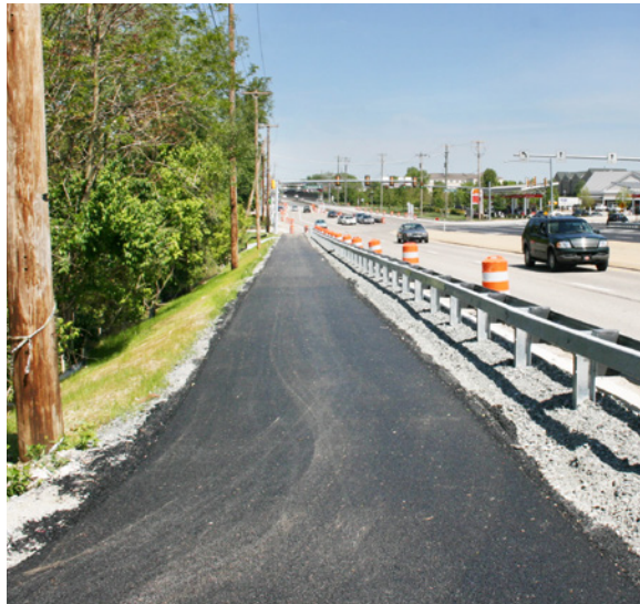
Chester Valley Trail sidepath along PA 29 in East Whiteland Township.
