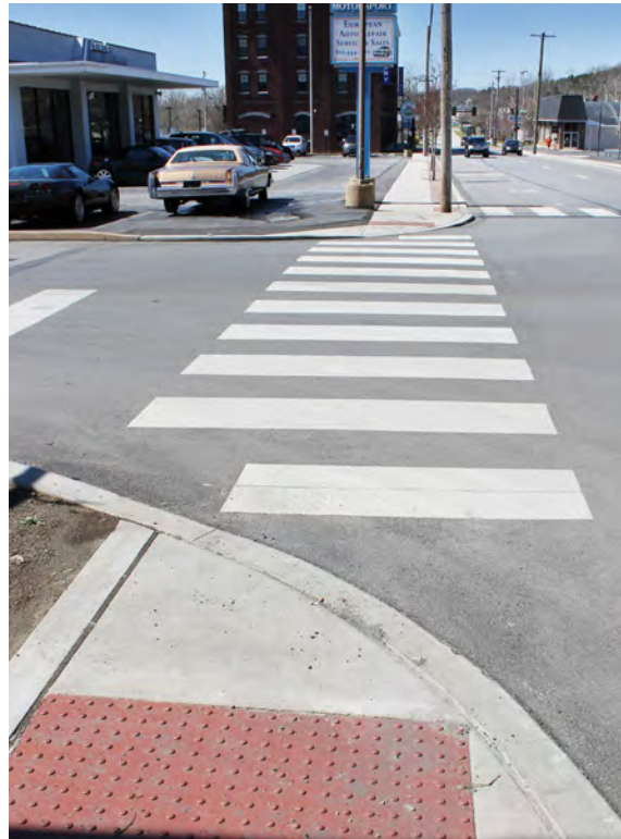
Example of ADA curb ramp and crosswalk.
