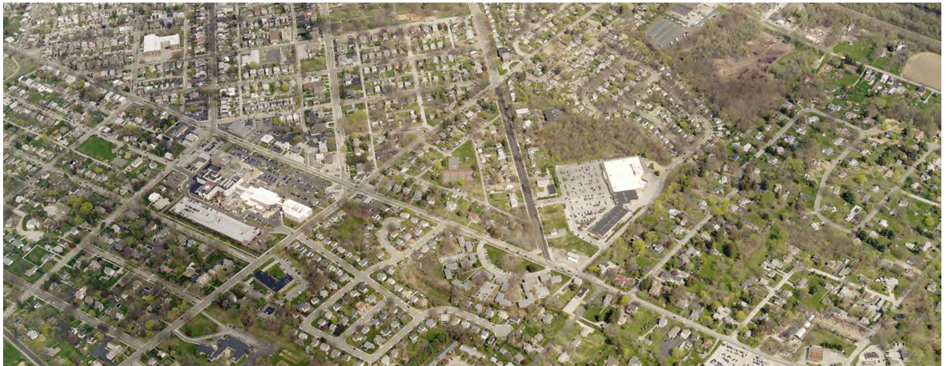
Aerial view of Phoenixville Borough, looking north. Source: Pictometry.
