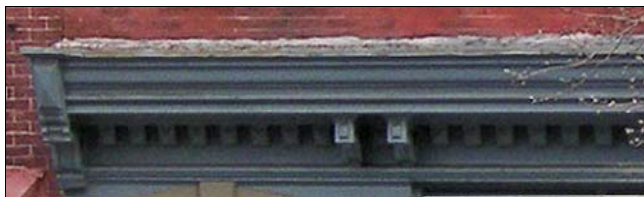
The bracketed cornice separates the storefront from the upper building levels.
