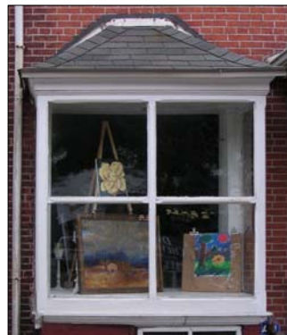
The bay window at this former residence is now used for a display.
