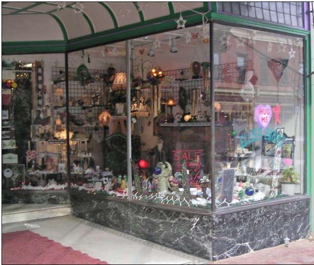
This storefront with a central recessed entry alcove has a large expanse of glazing allowing maximization of display area to attract potential customers. The storefront window apron is marble with patterned tile flooring.
