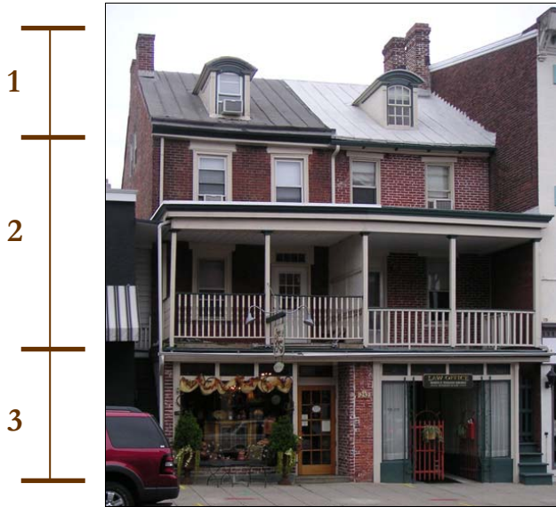
These residences have been modified for commercial purposes with the addition of storefronts at the ground level but retain their residential character above. Separate entrances for the residential and commercial uses are clearly distinguished and identifiable at the building to the right. Residential buildings converted for commercial uses are composed of three vertically stacked zones: 1. Roof and Building Cornice; 2. Upper Floors; 3. Storefronts.
