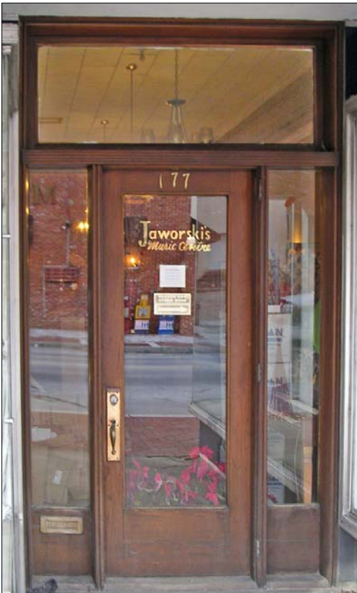
This wood entrance door system includes a central entry flanked by tall sidelights, all topped by a large transom window.
