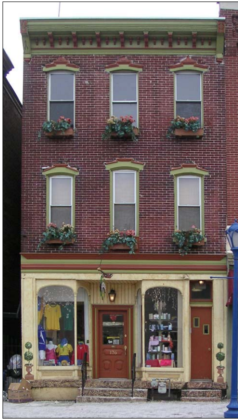
Commercial buildings are composed of three vertically stacked zones: 1. Ornamental Cornices; 2. Upper Floors; 3. Storefronts.
