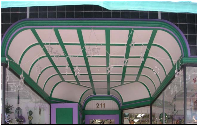
This arched entrance alcove ceiling has a simple geometric design at the ceiling that visually directs customers to the focal point of the central entrance door.
